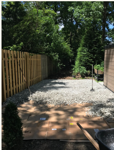
Service areas near the shed were stabilized with cardboard and stone.
