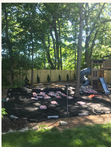
Staged materials and fabric defined the hardscape and play-surface zones.
