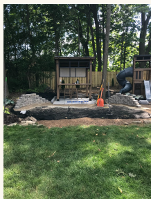
1. Wall blocks, sand, and fabric shaped the future fire-pit and lounge area.
