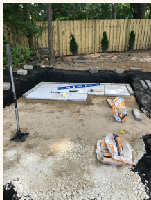
7. Base prep, leveling sand, and compaction set the foundation for the bar pad.
