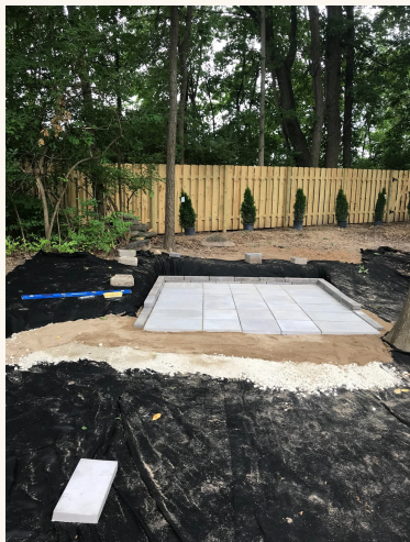
Pavers and border blocks locked in the footprint before the bar structure went up.
