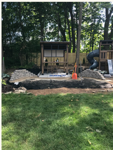
Wall blocks and staged base work began shaping the future lounge edge.
