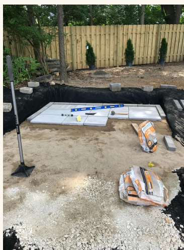
Leveling sand and base prep set the foundation for the paver pad.
