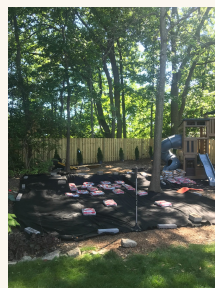
6. Fabric and staged material marked the hardscape and play-surface zones.
