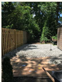
2. Service areas near the shed were stabilized with cardboard and stone.
