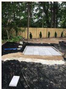
8. Pavers and border blocks locked in the footprint before the bar structure went up.
